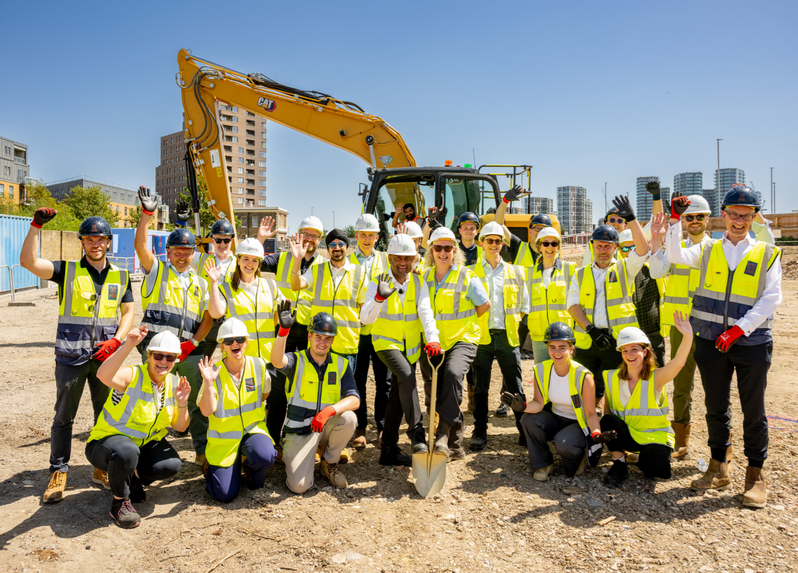
Above: Ground breaking at Pier Road in North Woolwich with Mayor Forhad Hussain.
